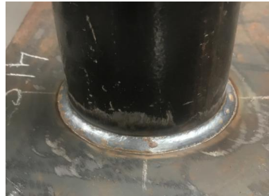
Pipe to Plate Fillet Weld
